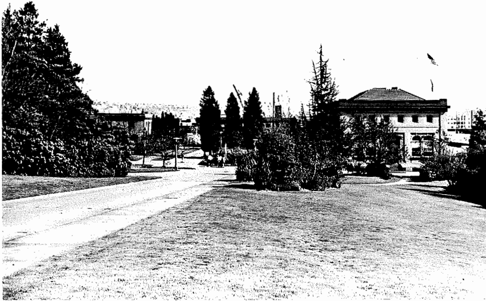
PHOTO 26: 1962. View east toward sub-area B5 and operations campus area from terraces. [1, 3, 4, 5, 12, 121/122, 309]. (LWSC 951)
