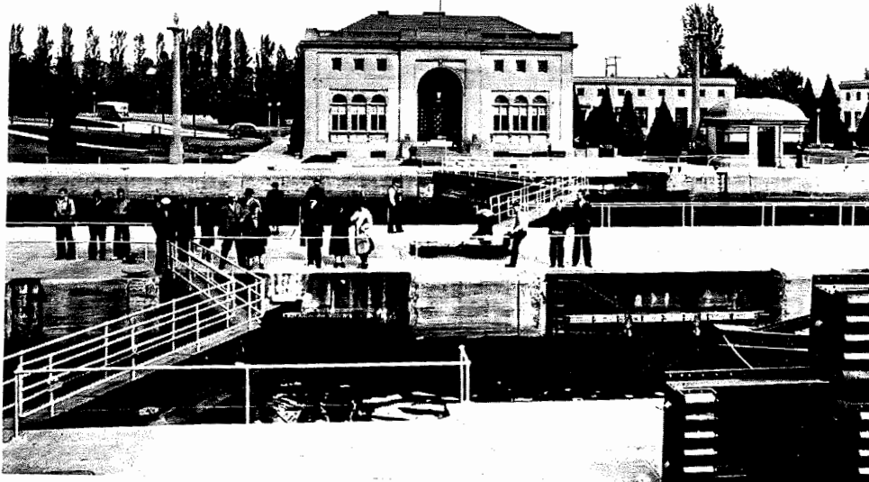
PHOTO 10: 1937. View north to Administration Building from spillway. [1, 2, 5, 12, 323, 324, 325, line of poplars in background, roped off lawn]. (P-2)
