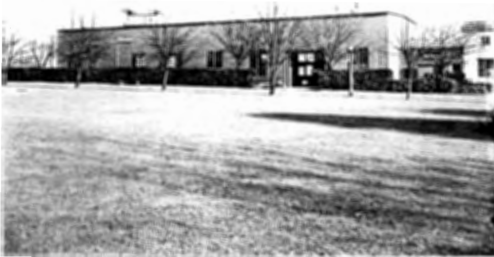
PHOTO 15: 1941. Warehouse #2 as seen across the lawn of sub-area B1. [125, original maples, clipped hedge]. (LWSC 90)
