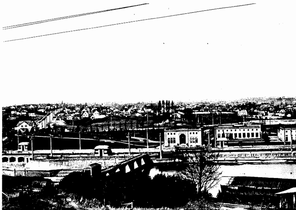
PHOTO 6: Locks grounds looking north from south side of canal. Outlines of Beds 325 and 326 can be seen in the right hand side of the photo showing that these beds were designed earlier than other garden history reports have stated. This photograph is mis-dated Dec. 1920. The size of specific trees and existence of Beds 325/326 date this sometime in late 1920's. (P-56)
