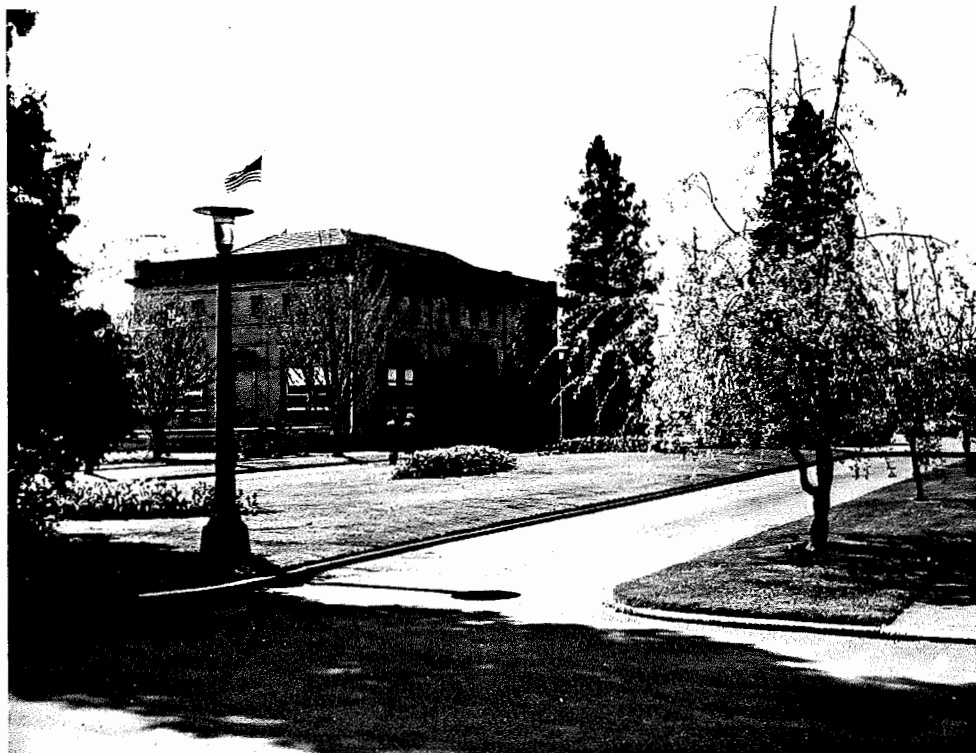
PHOTO 25: 1962. Operations campus area showing crescent shaped beds where rose garden now exists. [312, 316, 321, 323]. (LWSC 953)
