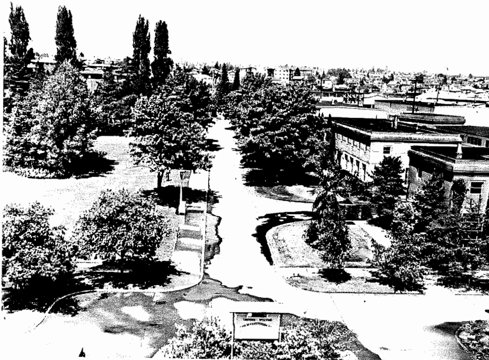
PHOTO 31: 1969. View north along entrance walk from the top of the Administration Bldg. [214, 305, 315]. (LWSC 1353)
